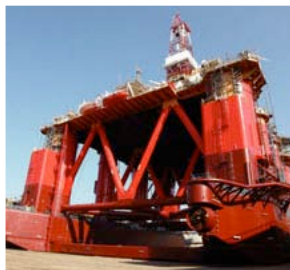
Deepdish工事後直後のHAKURYU-5
